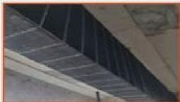
Micro-concreting work was done and all undulations were filled using the RELinforce \*\* EP Putty to provide a smooth surface, ready for CFRP application.
