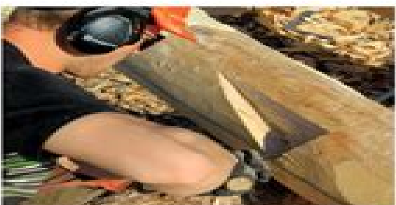
Figure 26: Cleaning out half of a joint. Note the lines on the top that are for tenon layout.
