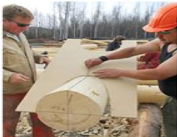
Figure 24: Dan and Hilko work on a truss in one of my hands-on courses. Note how the nail in hinge point helps position the flat surface that is used to trace the cut line onto the log. (This is sort of a portable C-jig, turned on its side.)
