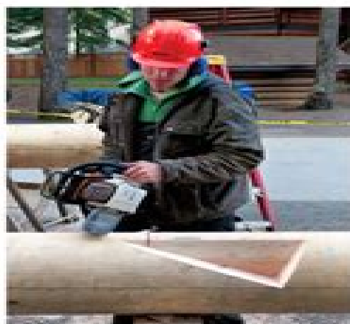
Figure 27: Left: Jordan chainsaws a tie beam joint where the rafter tail will be placed.
