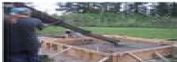
Excavating the shelter for the antenna. Building the concrete pad.
